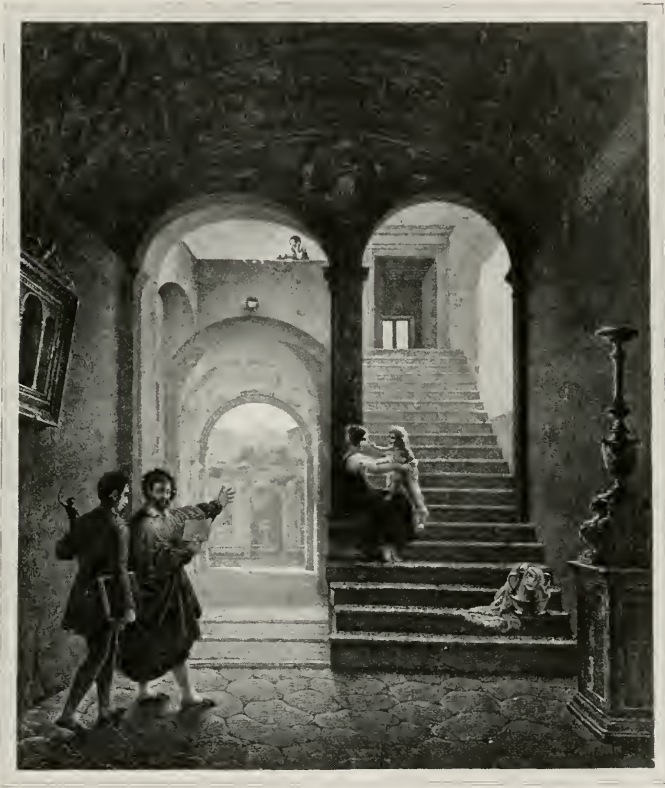
View of the vestibule of Michelangelo's house at the foot of the Capitol
